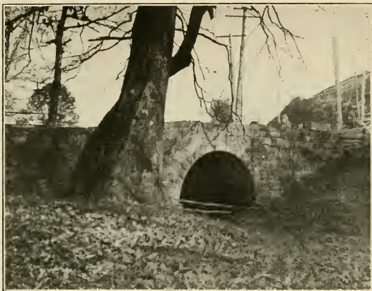
STONE CULVERT BRIDGE ACROSS FINK S RUN.
